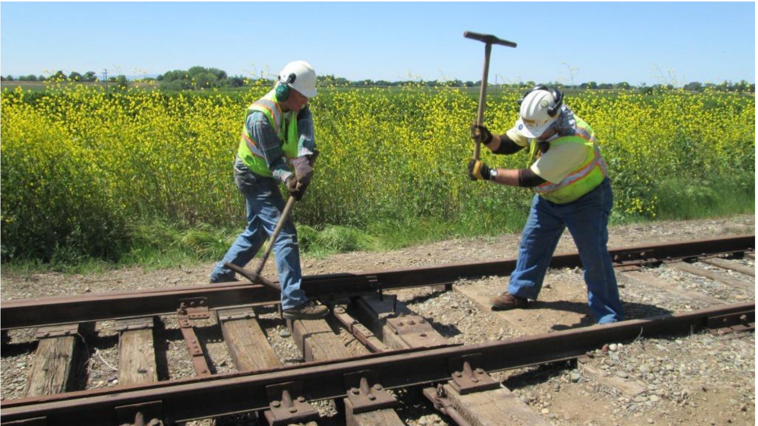
Now, Steve and Mike F. put on a show. They interpret old-fashion section-gang railroading by demonstrating tandem spike-driving
