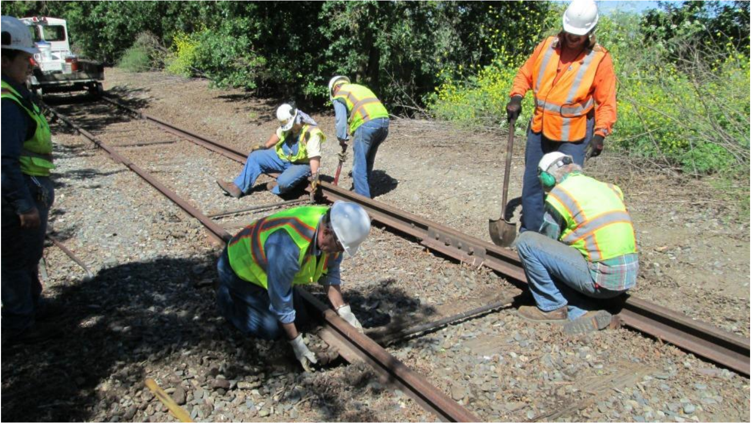
...And the clamps are tightened-down to push the rails apart
