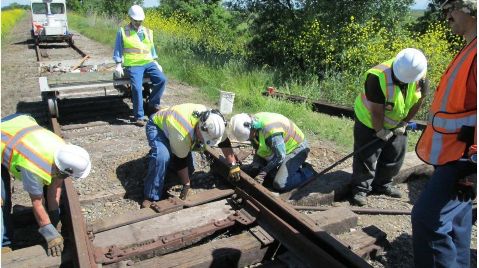
With the new head-block in position, it was time to get the gauge-plate in place. Clem, Mike F., and Steve work it onto the head-block as Anthony nips-up the rail so it can be slid underneath
