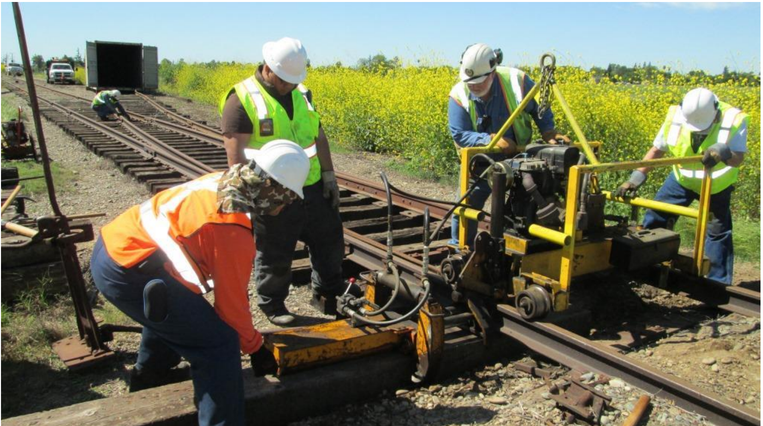
Because a head-block is much heavier than a tie, the section-gang machine had a bit of trouble letting-go after each pull. The clamps just weren't opening wide enough. So, Jose gives the pulling-ram a bit of a shimmy-shake to get it to release its hold on the head-block
