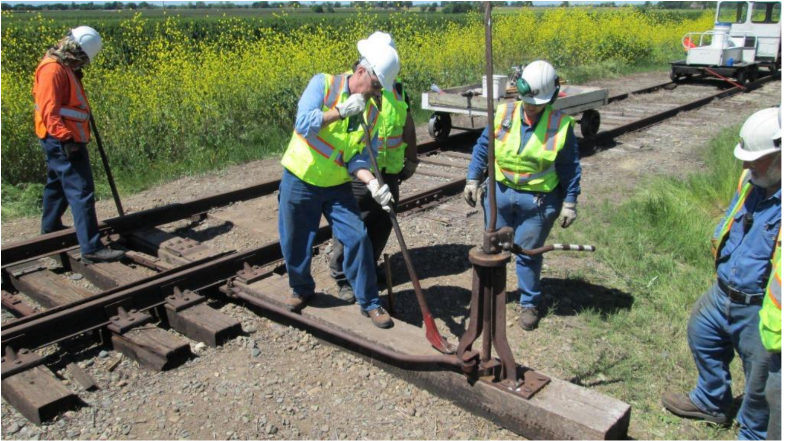
Ed pulls a spike on the switch-stand in order for it to be shifted slightly counter-clockwise
