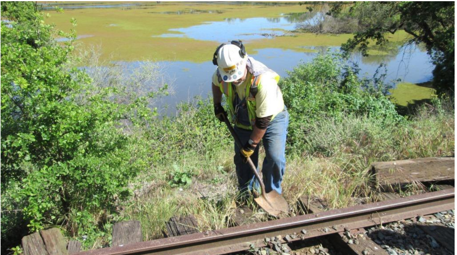
At the south approach to the fourth trestle, Mike F. digs under the rail to build a rail-stop
