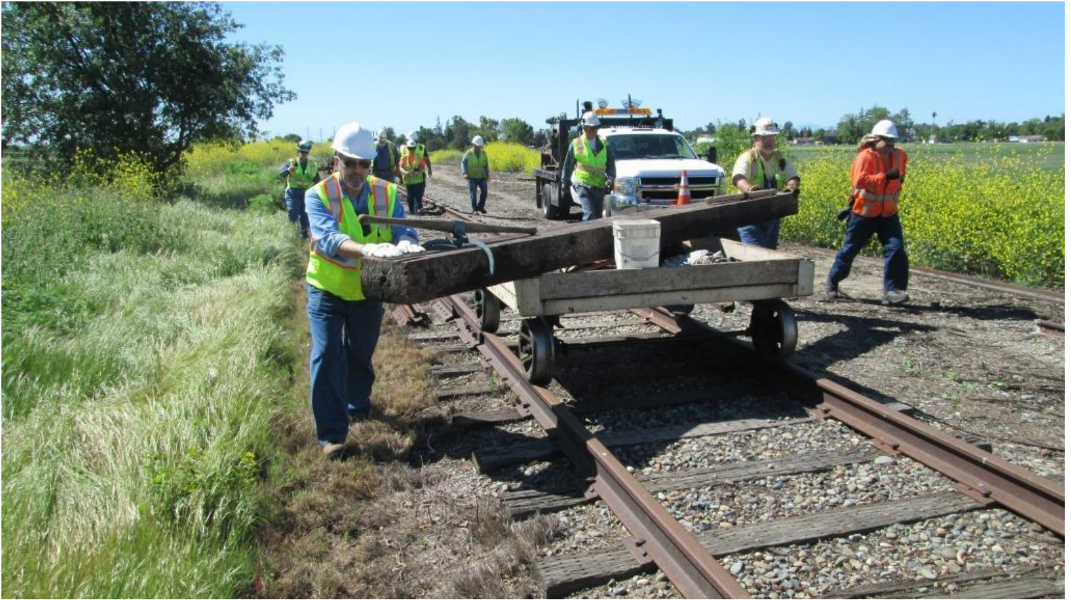
Ed and Mike F. roll the new head-block towards the switch
