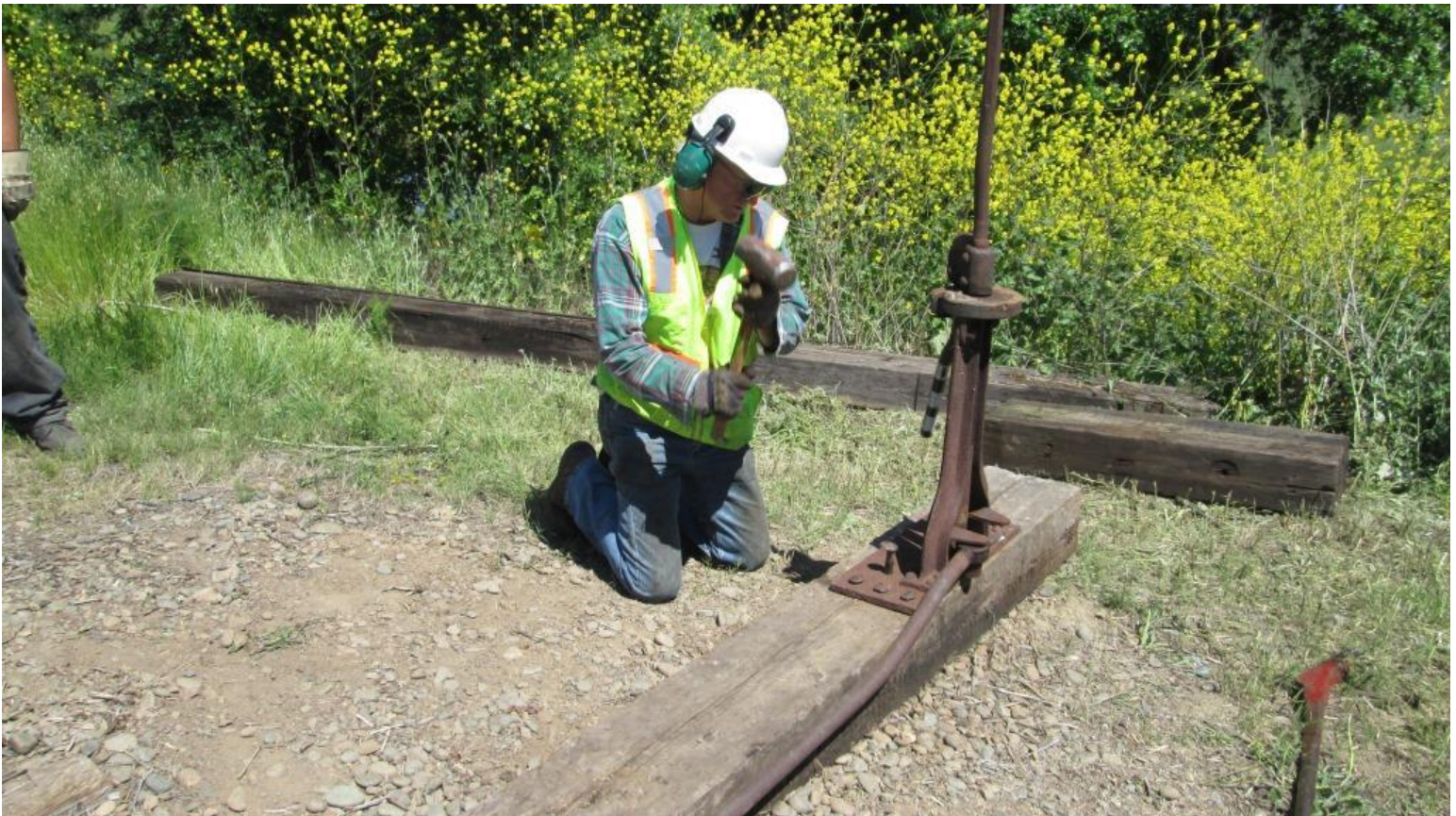
With everything now lined-up perfectly, Steve drives the final spike on the switch-stand
