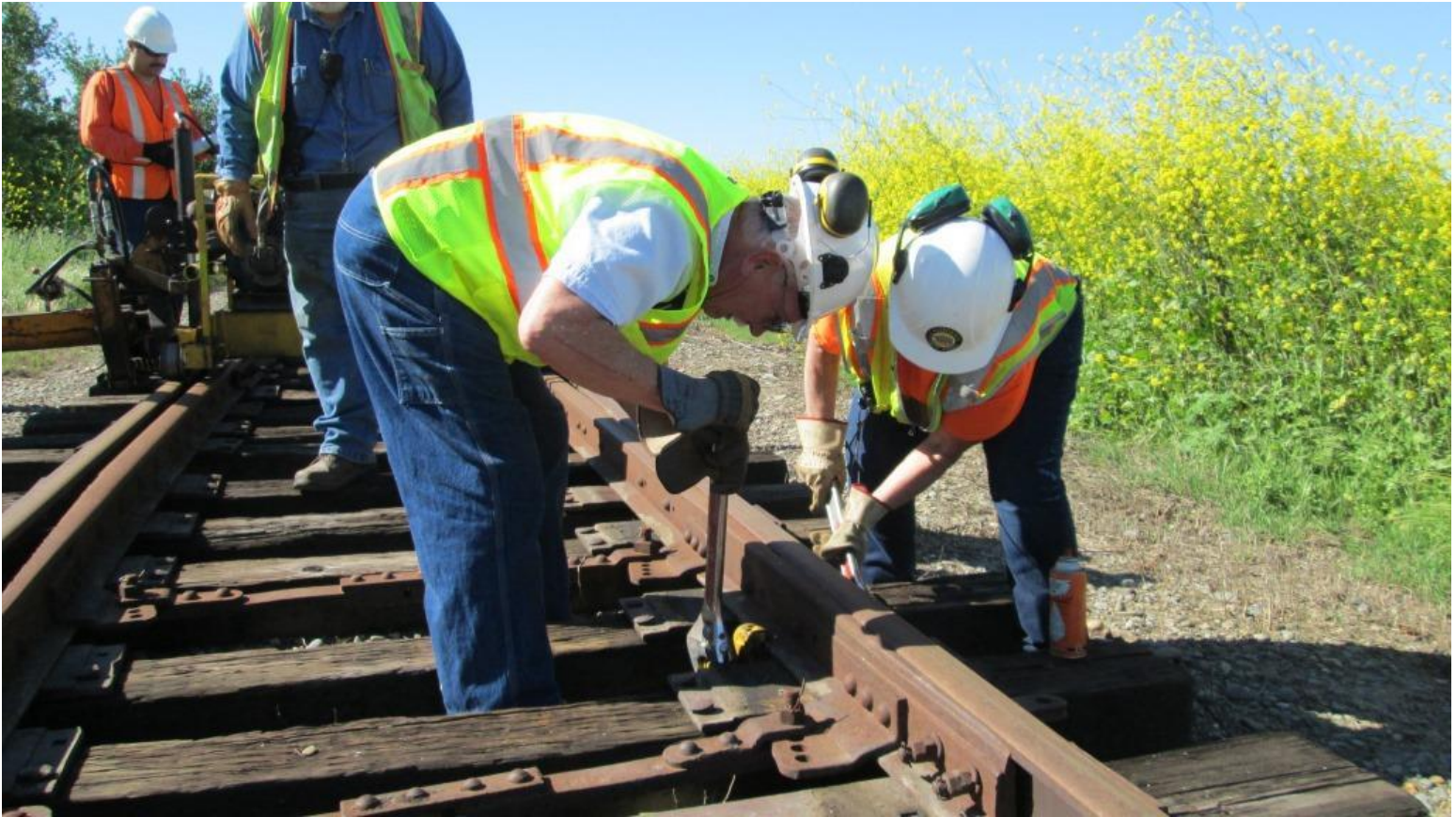
Clem and Pam tighten-down a clamp on the switch-points
