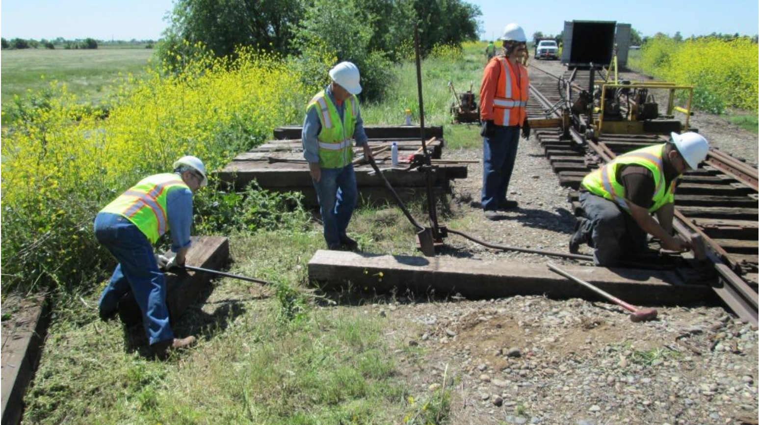
Anthony spikes down the gauge-bracket as Ed nips-up the head-block
