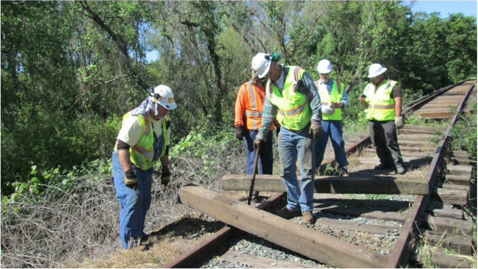
The Team brings in two ties to use as a rail-stop
