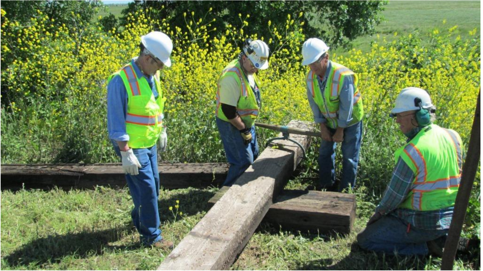
Mike F., and Mike T. line up the new head-block for insertion
