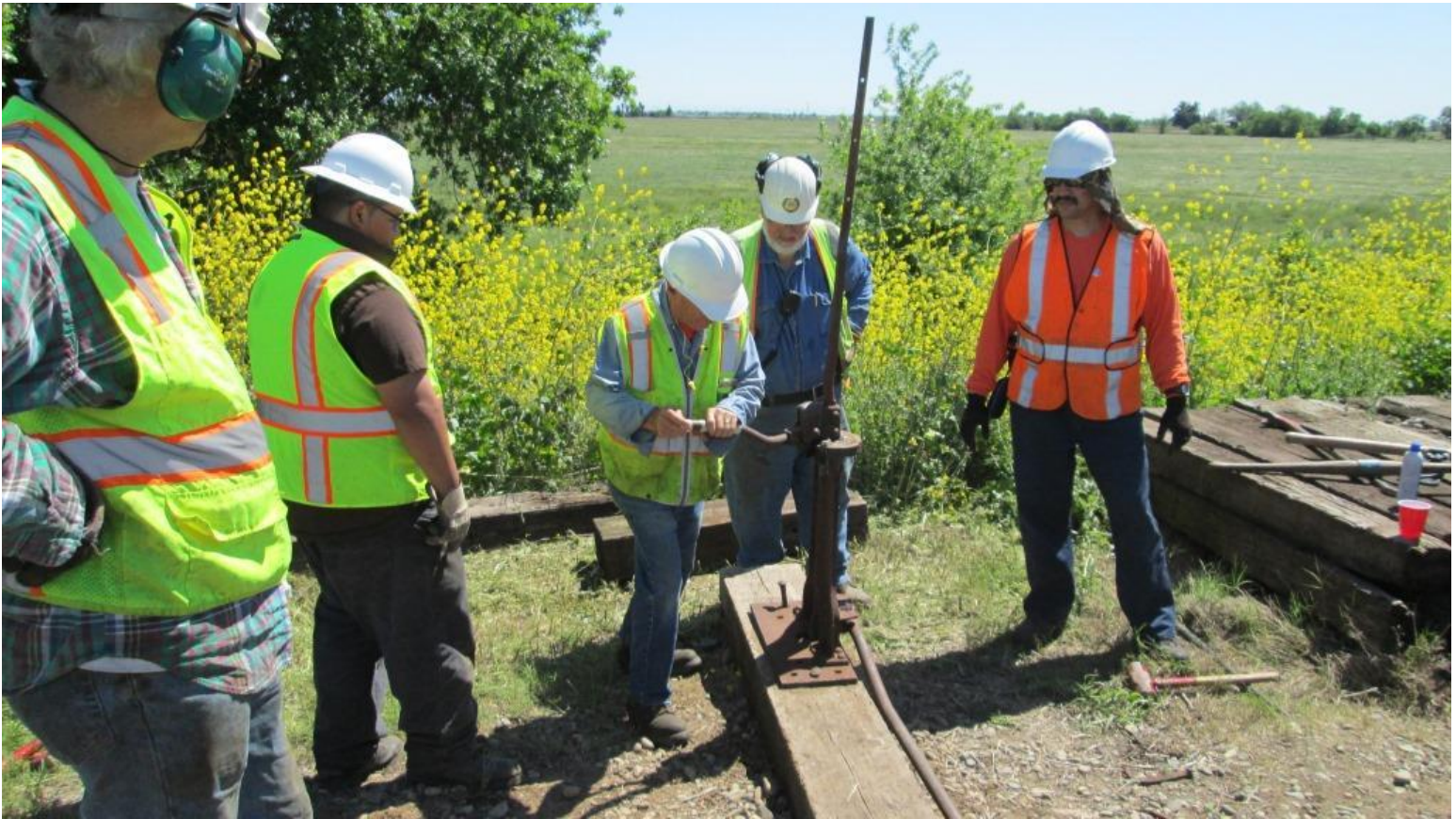
With the switch-stand now tacked-down, Mike T. tests it to check its position and make sure it's aligned properly
