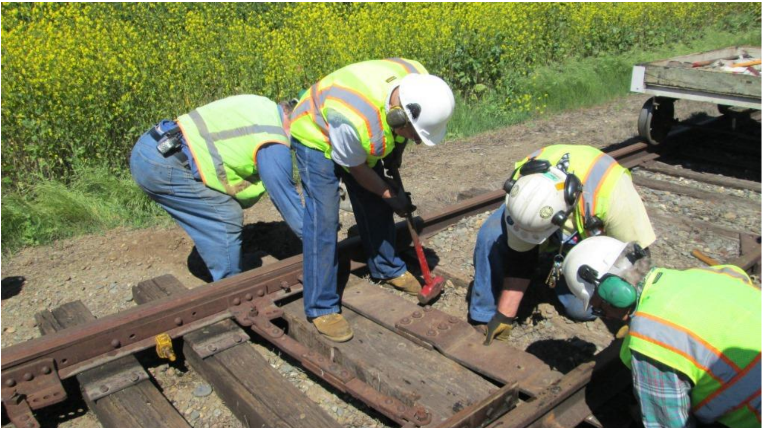
The gauge-plate was being a bit stubborn so, Clem uses the “ka-banger” tool to gives it a “ka-bang” into position
