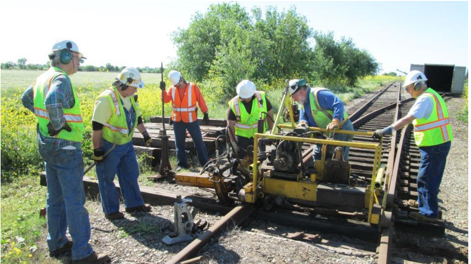
Frank operates the section-gang machine and pulls the old rotten head-block out from under the track
